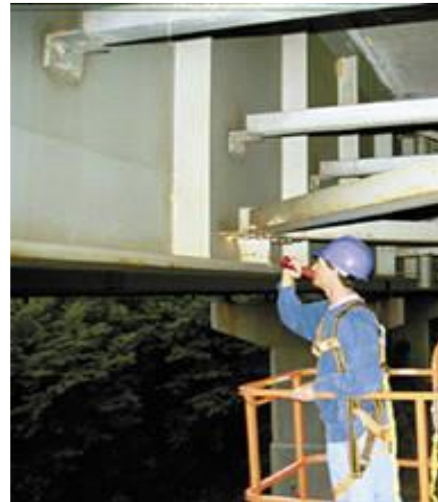
Inspection of a steel girder by visual inspection study
