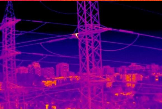
Electrical System Inspections
